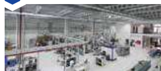
Expansion of production with new 13,000 m 2 production hall in Metzingen
