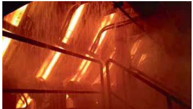
Secondary cooling zone of billet caster
