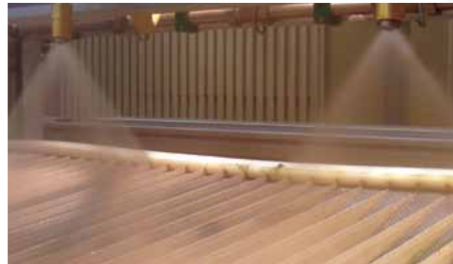
Liquid distribution measurement
