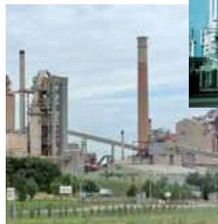
Cement and lime industry
