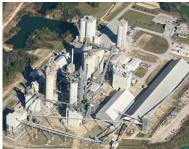
A new NH 3 injection system with the latest nozzle design by Lechler improved the performance of the SNCR system at a US cement plant
