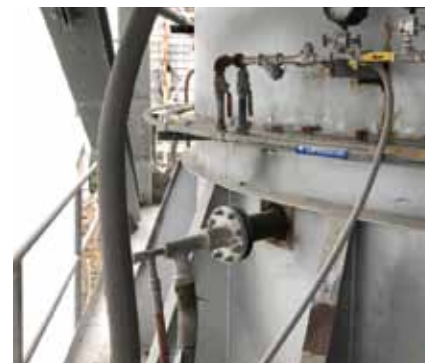
Figure 5: the new injection system in situ
